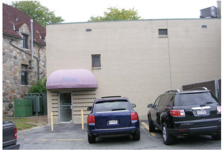
Rear parking with direct access to both levels of store
